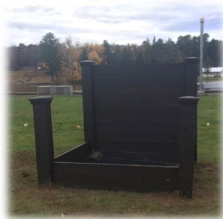
Invasive species disposal station at Chateaugay Lake constructed and installed by AWISP staff.
