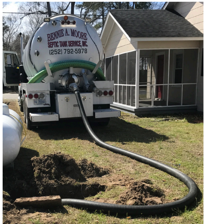
Septic tank pump out – photo from Benny A. Moore Septic Tank Service, Inc.
