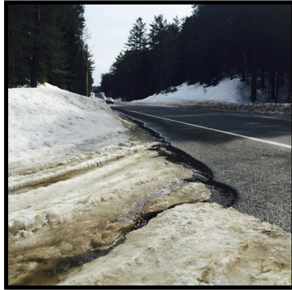
Image 9. Direct road salt runoff coming off of NYS RT 30 during a thawing event in the spring of 2015. The chloride concentration of this melt water was approaching 5,000 mg/L which is \frac{1}{4} the concentration of sea water.
